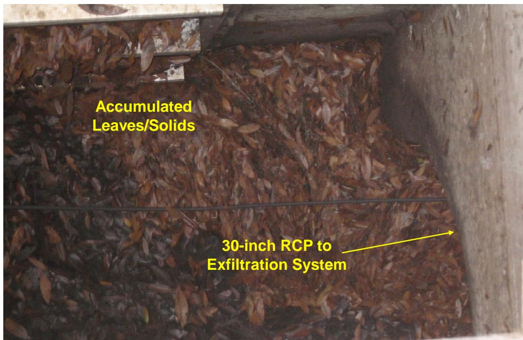
**Figure 2-7. Accumulation of Leaves Inside the Diversion Structure.**
